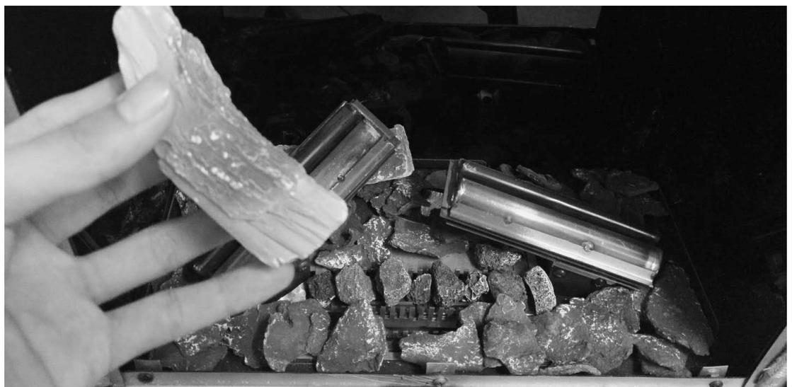
Place log D on the burner tray base at the back of the fire as shown in this picture.
