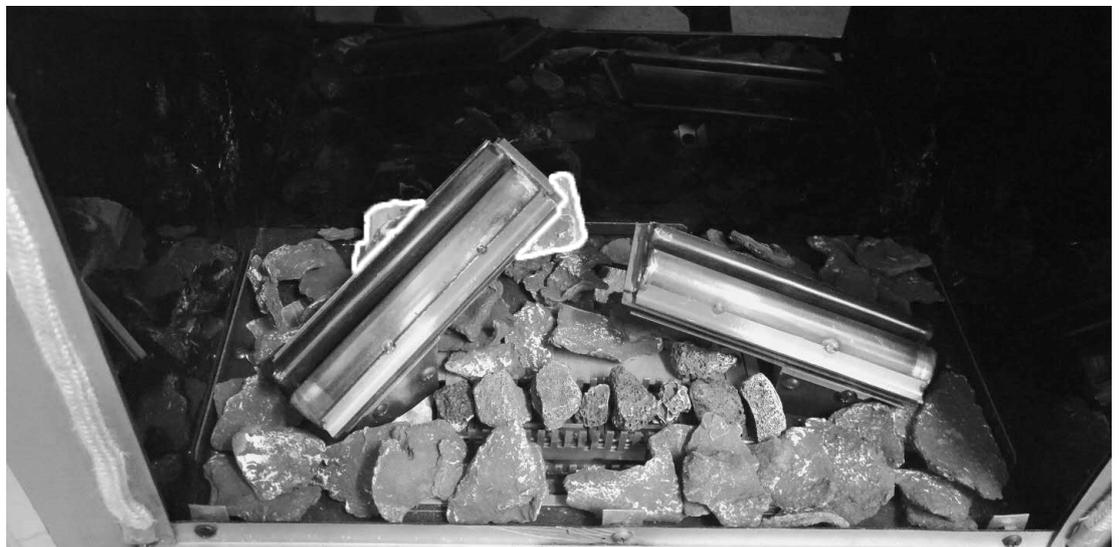
Identify and remove Log D from the ceramic packing carton. Note its orientation for installation in this picture.
